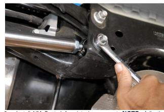
Install NM Control Arm into inner mount. NOTE: Adjusting flats on NM bar goes outward.
